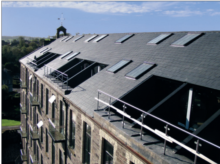
Figure 4 Conservation Centre Pivot Roof Windows
